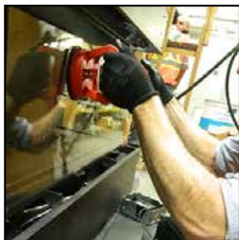
Handle glass with supplied vacuum clamps
