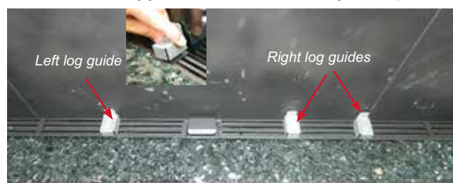
Log guides installed
