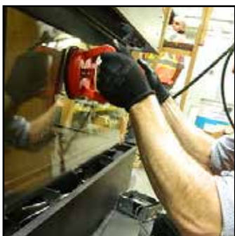
Handle glass with supplied vacuum clamps
