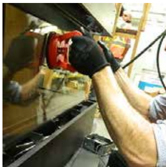
Handle glass with supplied vacuum clamps
