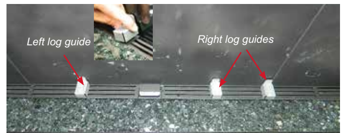
Log guides installed
