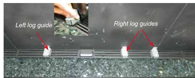
Log guides installed
