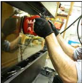
Handle glass with supplied vacuum clamps
