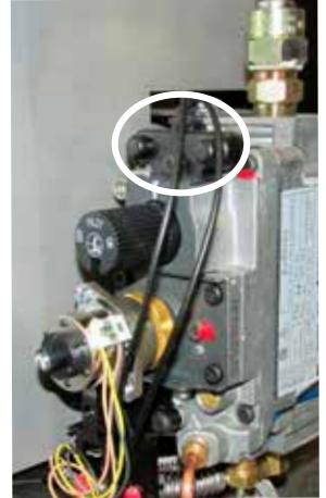
DC Sparker Wires
