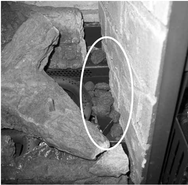
Right side of Burner
