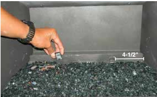
Log bracket install
