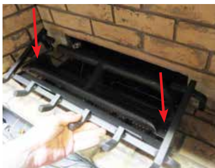
Diagram 1: Remove the left and right screws.
