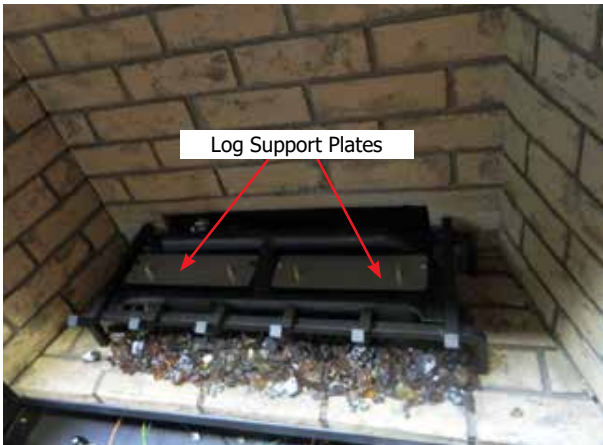
Diagram 6—Log support plates installed
