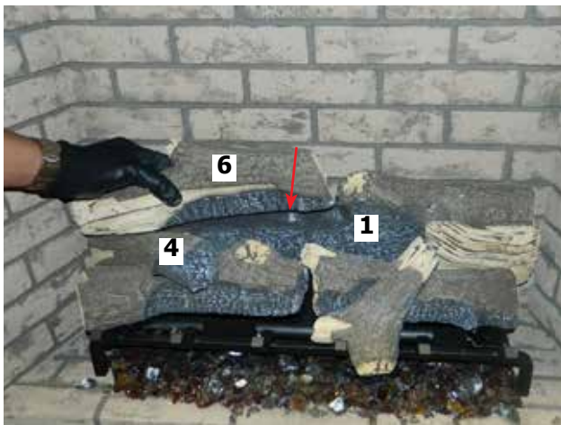
Diagram 12—Install Log 6
