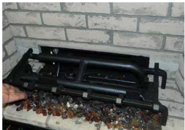
Diagram 4—Install Vermiculite + Lava
