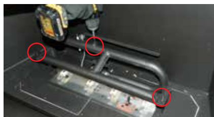
Diagram 2: Slide burner assembly to the right—then remove.
