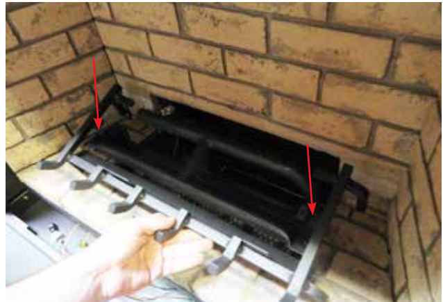
Diagram 2—Log Grate Install
