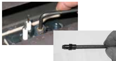
Diagram 2: Slide burner assembly to the right—then remove.
