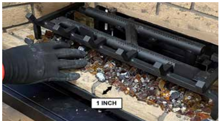
Diagram 4-Install Vermiculite + Lava Warning: Glass crystals must be placed at least 1" away from the front edge of the unit.
