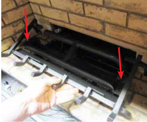
Diagram 1: Remove the left and right screws.
