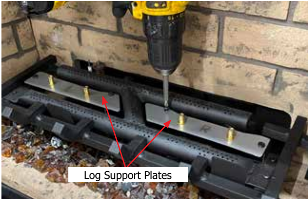
Diagram 5-Install Log support plate installation
