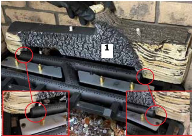
Diagram 6-Log 1 installation
