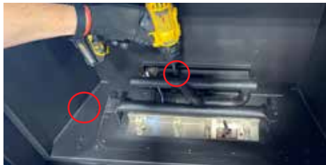
Diagram 2: Slide burner assembly to the right—then remove.
