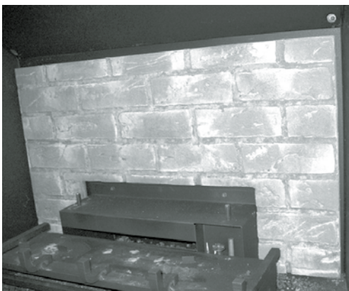
Back Panel Installed
