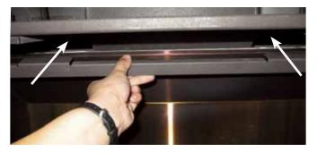
Top panel bracket shown installed with Stainless Steel Panels
