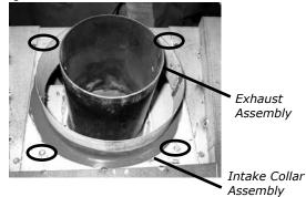
From the outside rear of the firebox: install the intake cover plate with 4 - 1/4" x 1/2" screws. Ensure all screws are tight, but do not over tighten. All 4 screws must be used.
