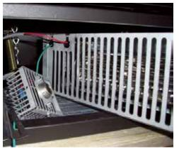
Lift the fan housing upwards and slip it over the two mounting studs. (use of dish soap will help the rubber grommets slide down over the pins)
