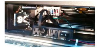
11. Plug in the fan power cord to the Fan Control Module into the outlet marked "Fan". Plug the FCM-COM wire from the remote control wiring harness into the location on the Fan Control Module marked "COM". Turn the switch on the Fan Control Module to the ON position. ON is to the left. The "O" is the off position
