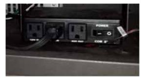
8) Plug fan power cord into the Fan Control Module (FCM) then plug in the FCM. The switch is on when pushed to the left. (Shown in OFF position above)
