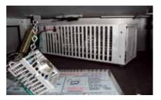
9) Slide the thermodisc/cover assembly onto the bracket clip on the left underside of the firebox. Ensure that no wires will touch hot surfaces.
