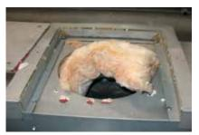
9. From the outside back of the firebox: locate the insulation deflector and bend completely upwards flat against the back of firebox.
