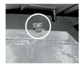
6) Slide the top brick panel under the left or right side panel (which ever is installed first - right side panel shown here) and back brick panel, use care not to damage panel.
