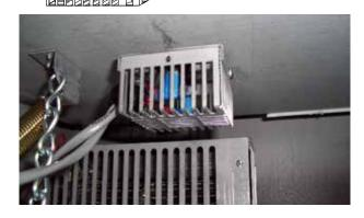
**10.** Install the Fan Control Module (FCM) on to the left side base of the unit and plug in to electrical receptacle in unit as shown.
