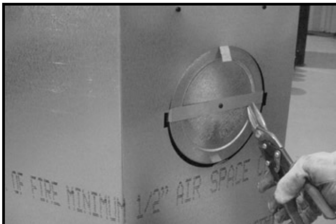
Figure 6.8 (Generic Fireplace Shown) Cut the metal retaining band and fold the sides out.
