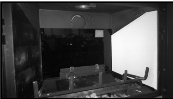
Figure 2. Install Rear Glass Panel
