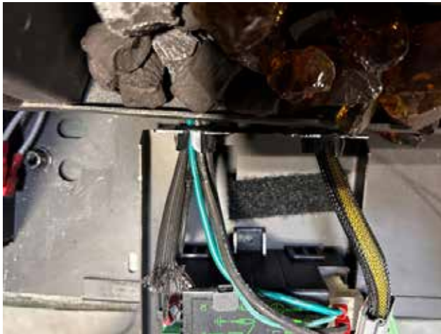
Diagram 7 Velcro affixed to IFC Tray
