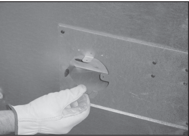
Figure 3.19 Bending Tabs on Outside Air Kit Collar
