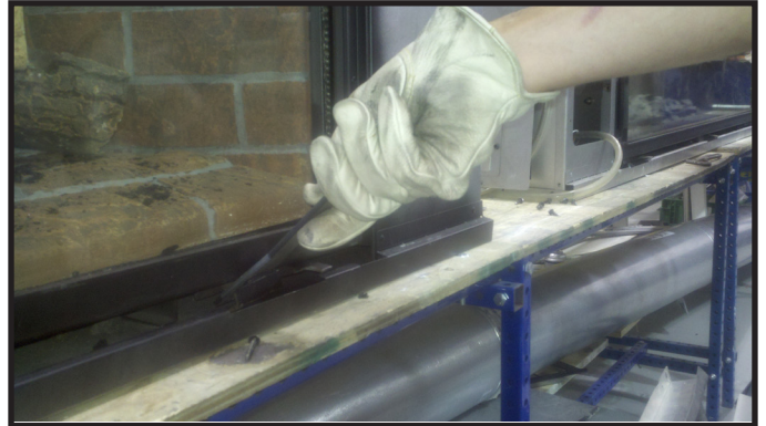
Figure 11.3. Inserting Glass Clip Tool
