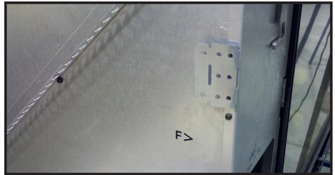
Figure 6.4 Side Nailing Tab in Shipping Position
