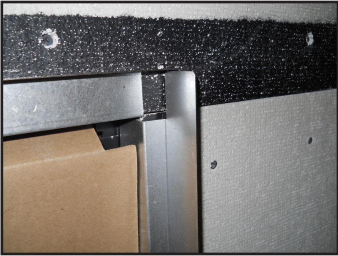
Figure 10.5 Finishing Template Bends
