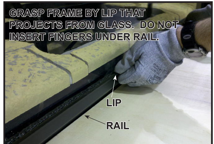
Figure 11.6. Installing Glass
