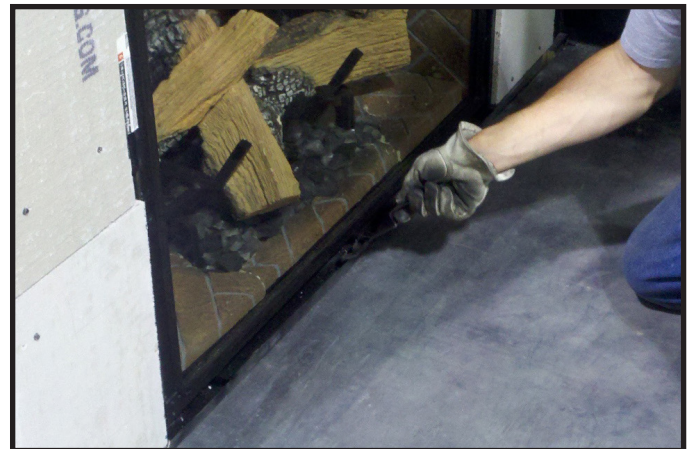
Figure 11.8. Securing Bottom Glass Clips
