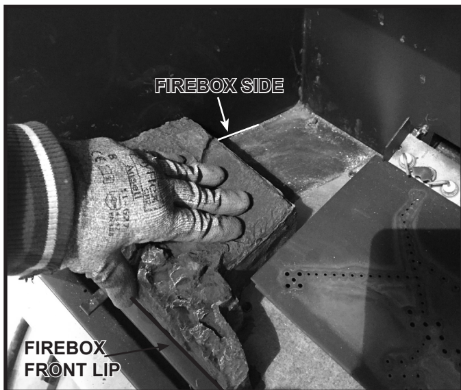
Figure 11.2 Install Left Hearth Component
