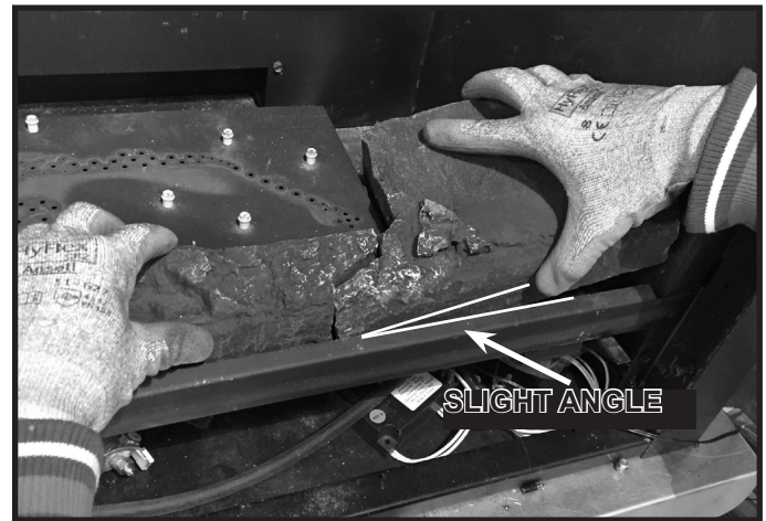
Figure 11.4 Lift Center Hearth Component While Placing Right Hearth Component
