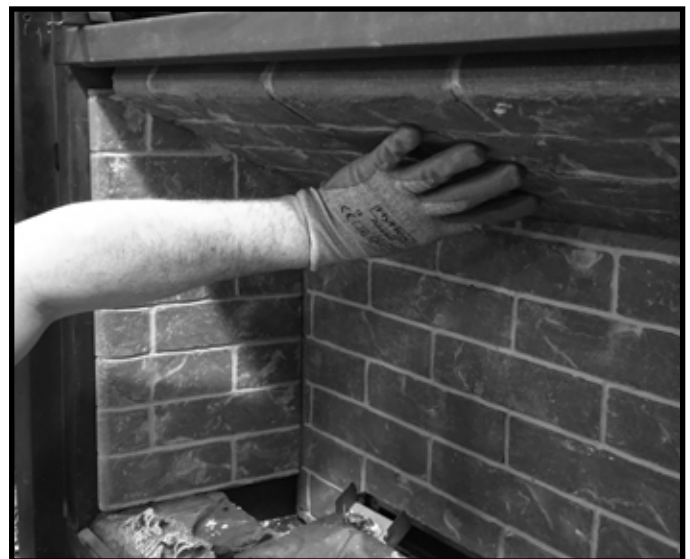
Figure 11.5 Install Right Refractory Panel
