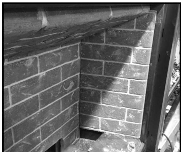
Figure 11.6 Right Refractory Panel Installed
