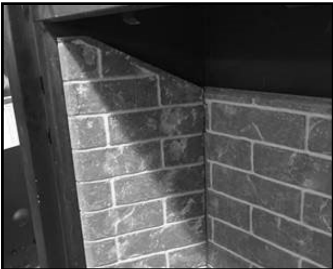
Figure 11.3 Install Left Refractory Panel
