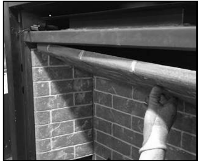
Figure 11.4 Install Top Refractory Panel
