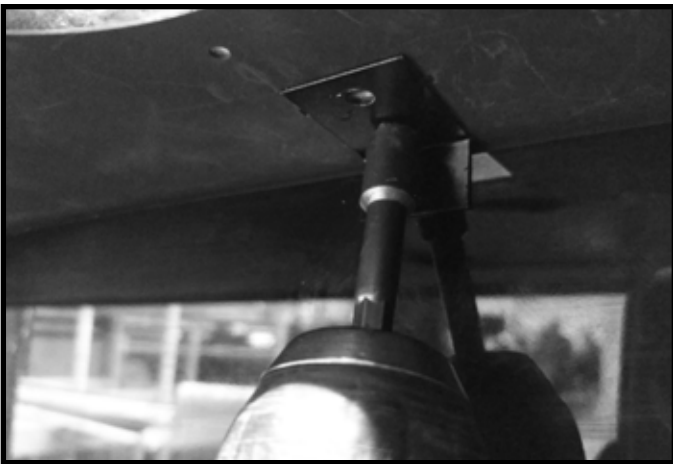
Figure 3 Retaining Bracket Installation - Back
