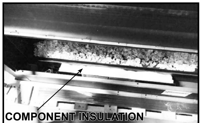
Figure 11.3 Component Insulation Location
