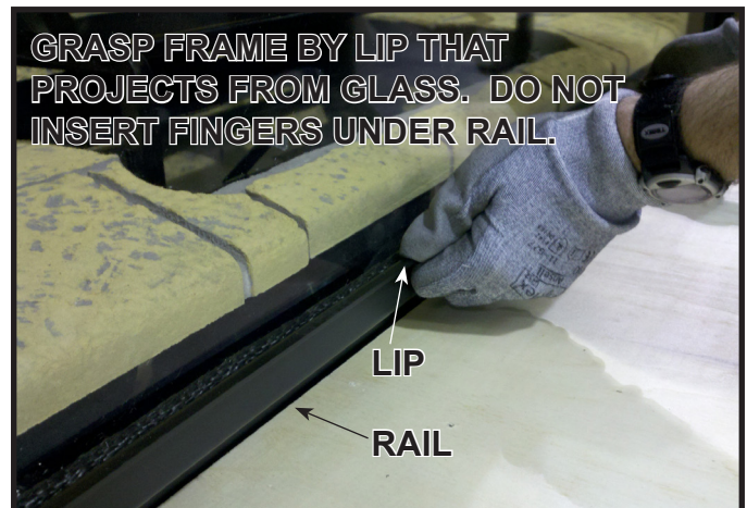
Figure 11.6. Installing Glass
