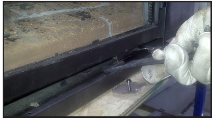
Figure 11.2. Glass Clip Tool Location
