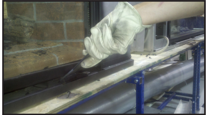
Figure 11.3. Inserting Glass Clip Tool
