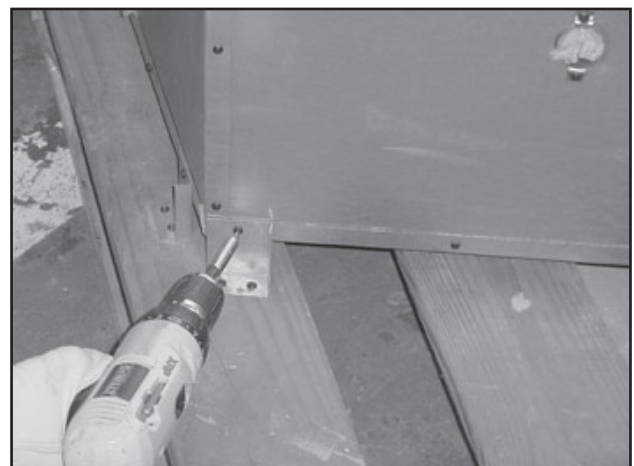
Figure 3.12 Removing Shipping Brackets
