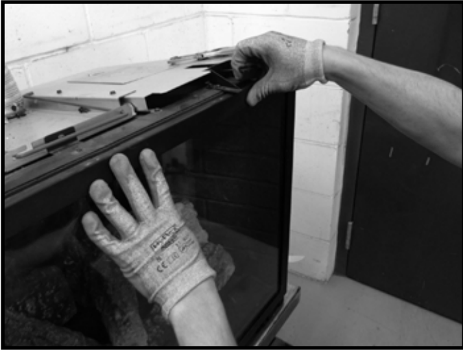
Figure 11.4 Release Glass Latches One at a Time
