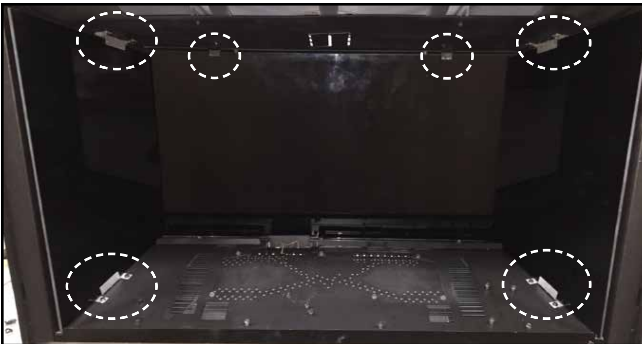
Figure 6 All Glass Panels Installed
