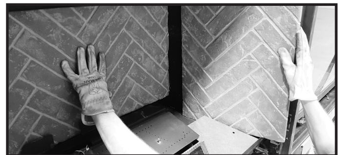
Figure 11.3 Install Side Refractory Panel (Right Side Shown)
